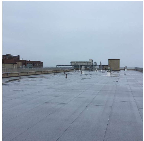
Roof 1 - Southeast view
