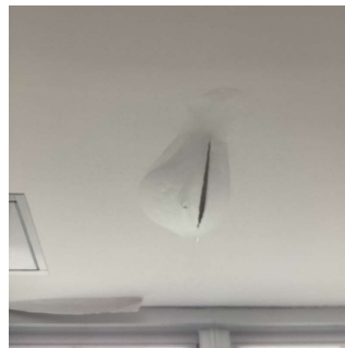
Roof 4 - 1st Floor Kitchen Storage, also Roof 1 - Stair D/3, Corridor near Stair D/3, Corridor near Room 319, Corridor near Room 313, Corridor near Room 301, Roof 2 - Gymnasium
