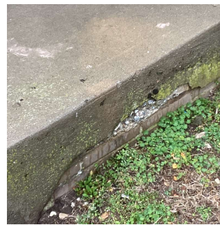
Facade A No violations recorded.
