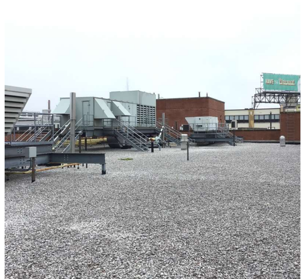
Roof 1 - Southeast view
