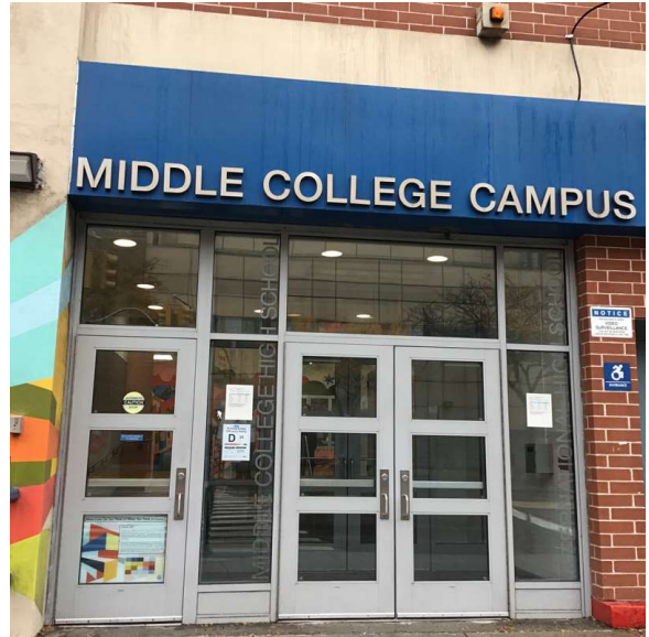
Facade A - Van Dam Street
