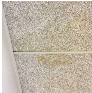
Roof 3 - Corridor near Room 258, also Room 256, Roof 1 - Room 221
