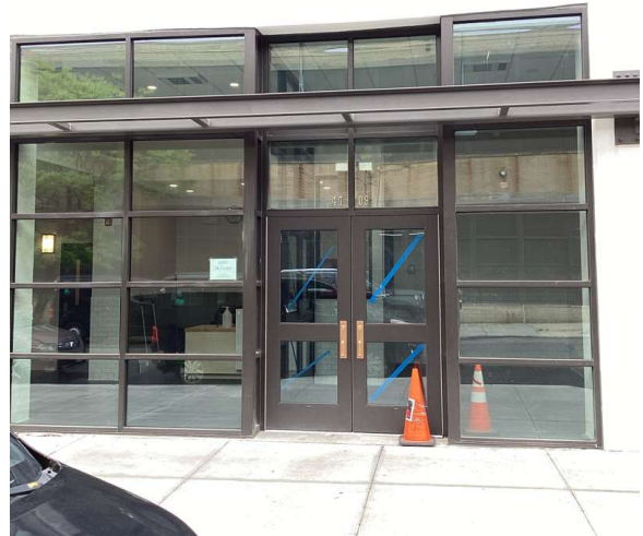
Facade A - 36th Street
