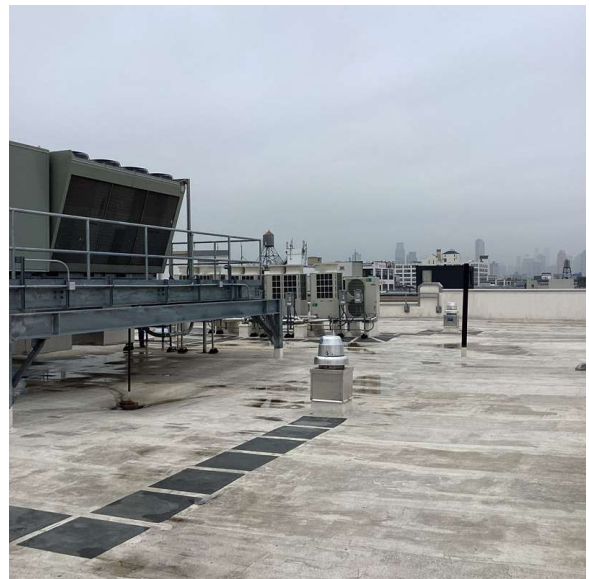
Roof 1 - West View
