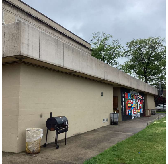
Corner of Facade A and Facade B - Southwest view
