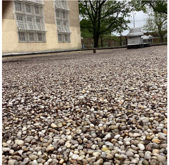
Roof 1 - Southwest view
