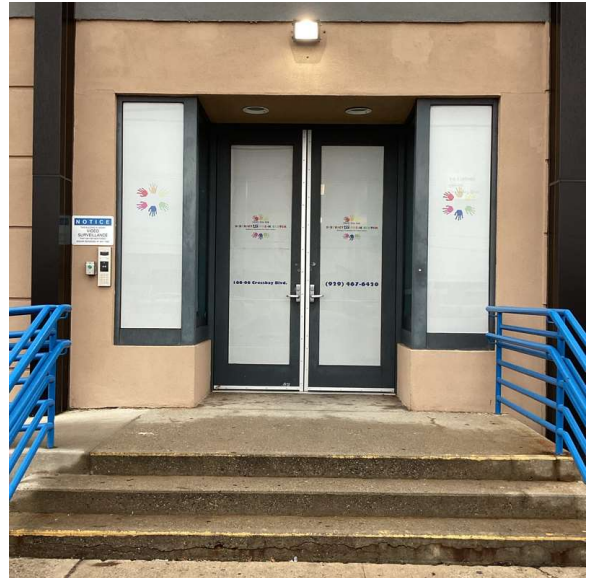
Facade A - Cross Bay Boulevard
