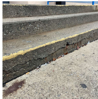
Facade A No violations recorded.
