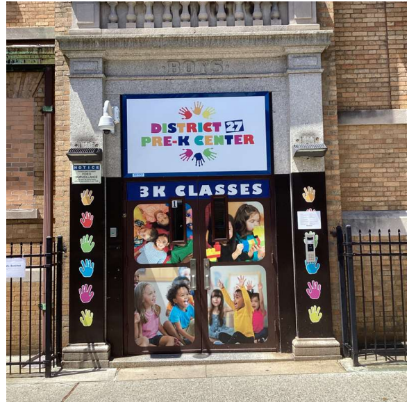
Facade A - 88th Street
