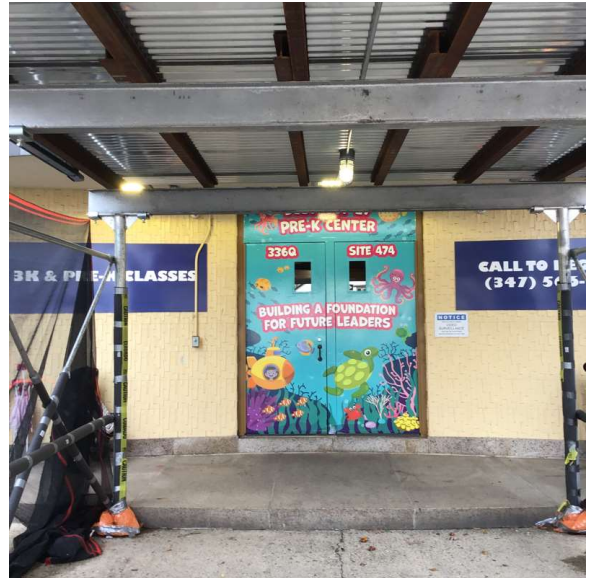
Facade A - 105th Street
