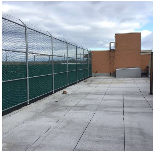
Roof 1 - Northeast view
