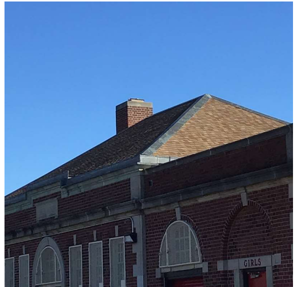
Roof 1 - Southeast view
