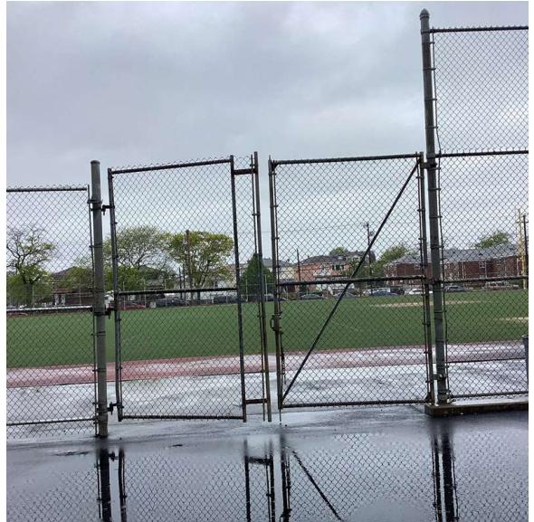
Main School Backyard - Southwest View
