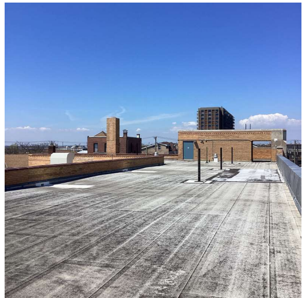
Roof 1 - Northwest view
