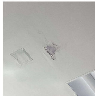
Roof 2 - Multipurpose Room, also Room 111, Corridor near Room 115
