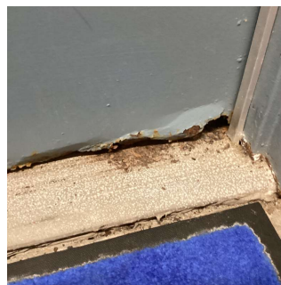
Facade B No violations recorded.
