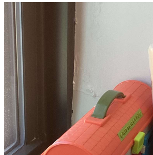
Facade D - Room 210 (two locations) also Facade A - Room 206 No violations recorded.
