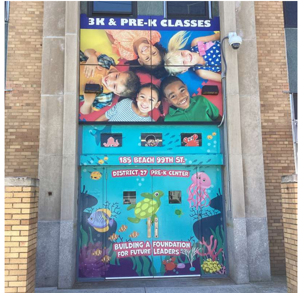
Facade A - Beach 99th Street
