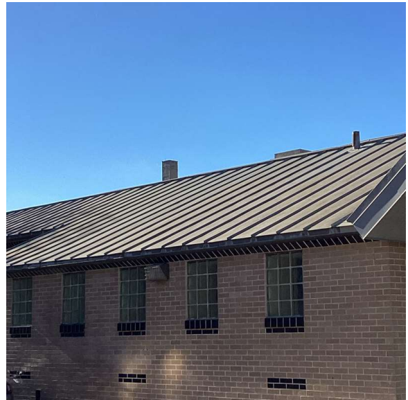
Roof 1 - South View
