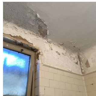
Roof 4 - Girls Toilet Room
