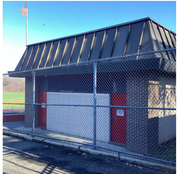
Roof 2 - Northeast View
