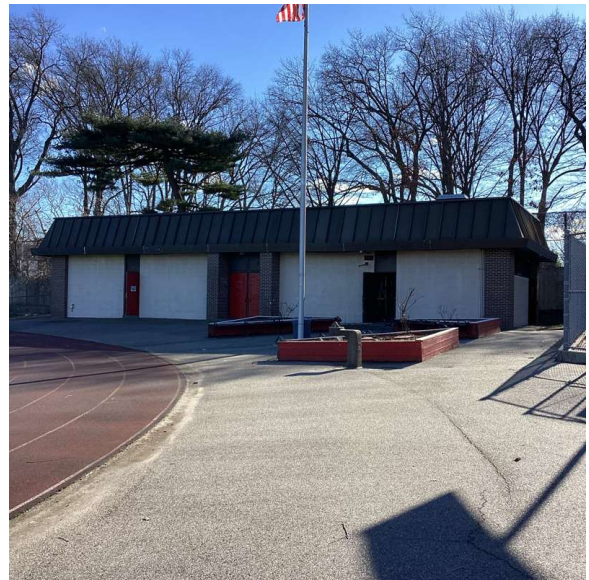
Field House 1 - Southeast View
