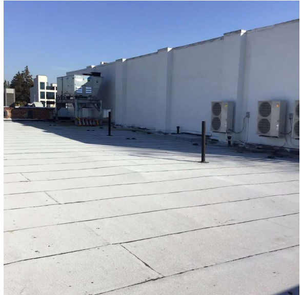
Roof 1 - East View
