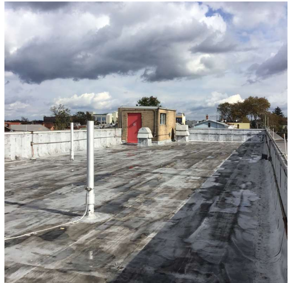
Roof 2 - Southwest View
