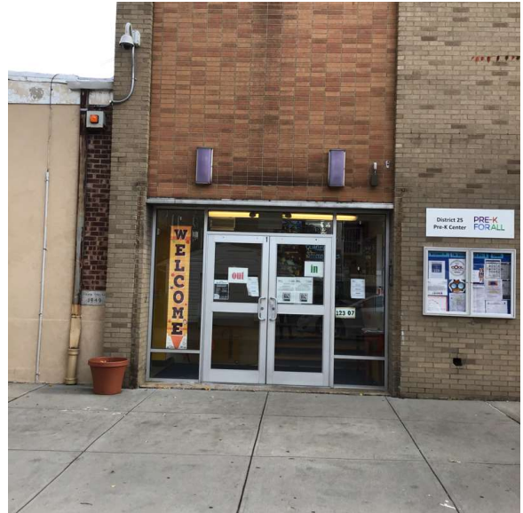
Facade A - 123rd Street
