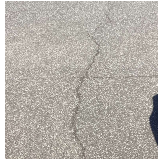
Tennis Courts No violations recorded.
