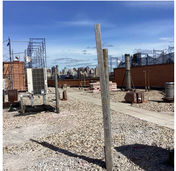
Roof 1 - Northeast view
