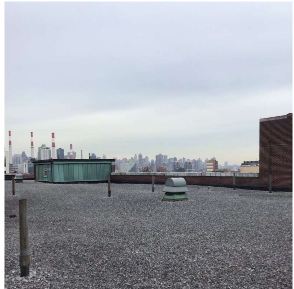
Roof 1 - South View
