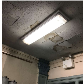
Corridor near Exit 9 - Vestibule
