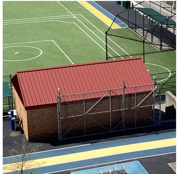
Roof 1 - Southwest View
