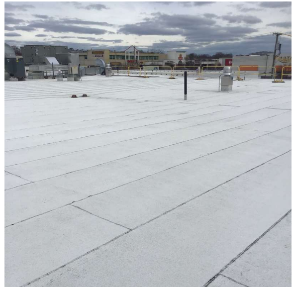
Roof 1 - Northeast View
