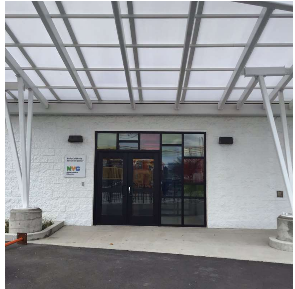
Facade A - 132nd Street
