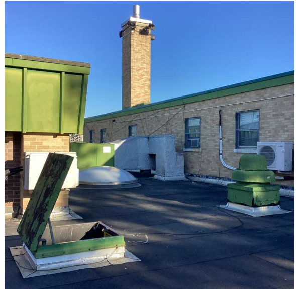
Roof 1 - North View
