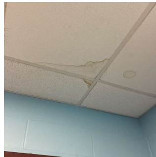
Roof 1 - Room 103 (Roof 1 - Room 104 similar)
