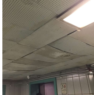
Corridor near Room B03
