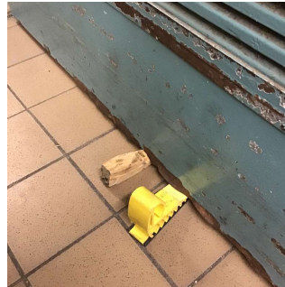
Storage Room Near Lockers
