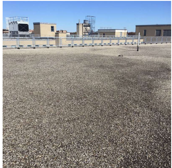
Roof 1 - Northwest View
