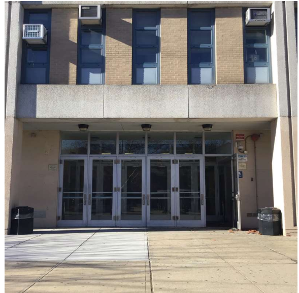
Facade A - 223rd Street
