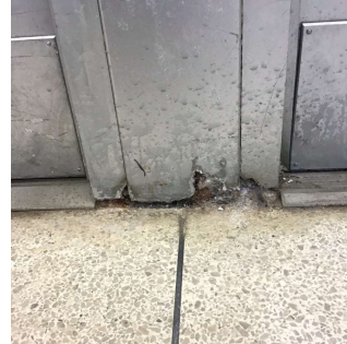
Facade C - Exit 14
