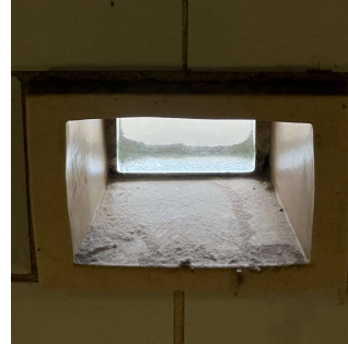
Facade B - Stair C/2
