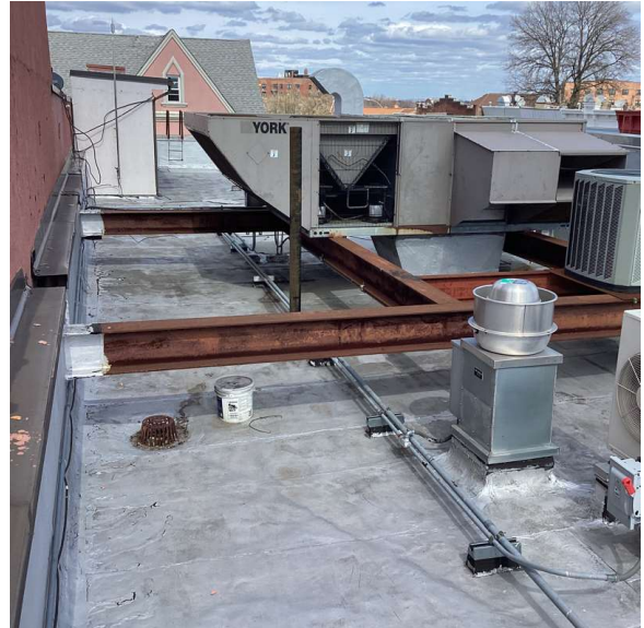
Roof 1 - North View
