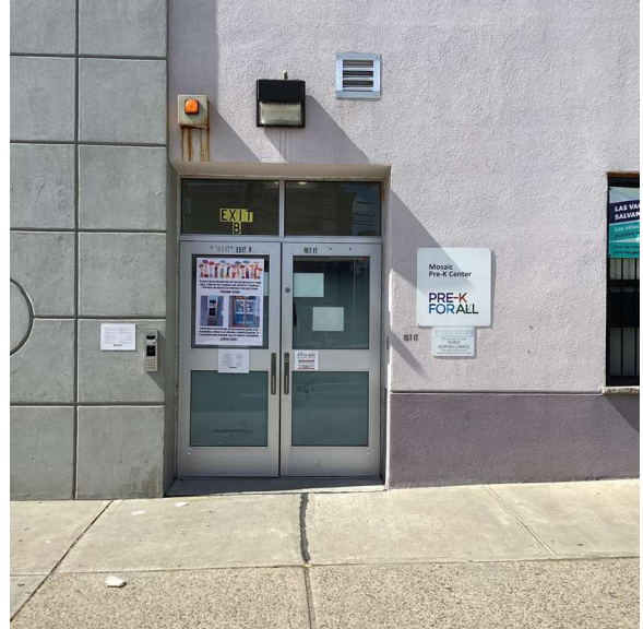
Facade A - 108th Street
