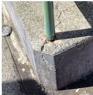
Facade A No violations recorded.
