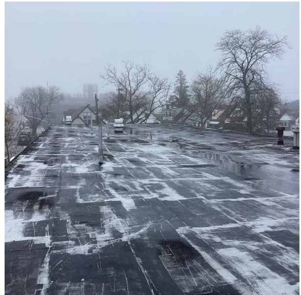
Roof 1 - North View
