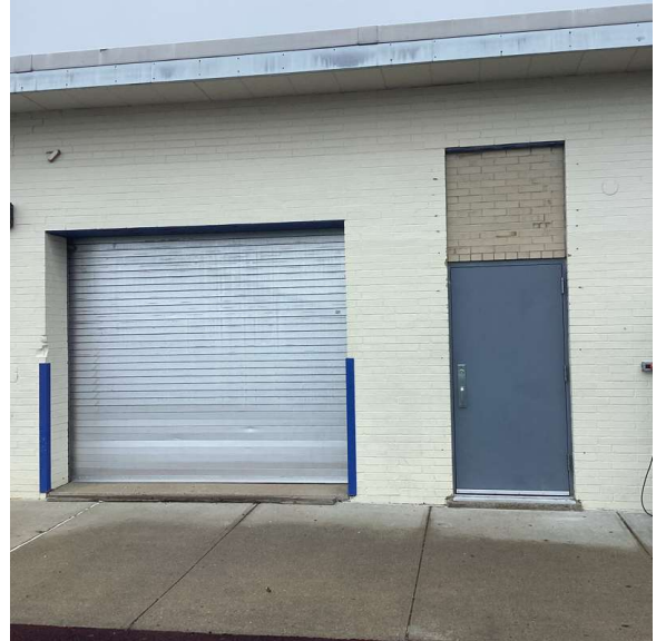
Facade A - Fieldhouse
