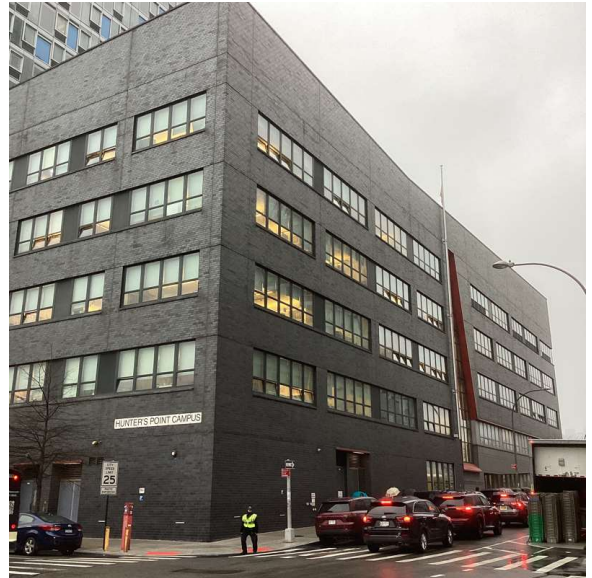
Corner of 51st Avenue and Center Boulevard - Southeast view
