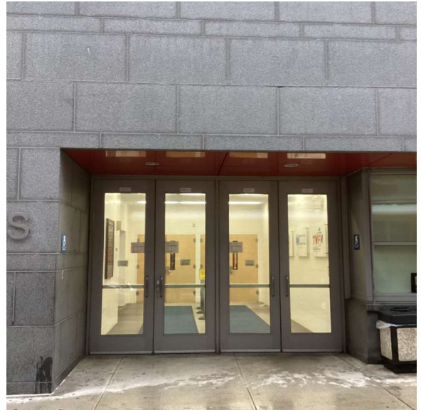
Facade A - 51st Avenue
