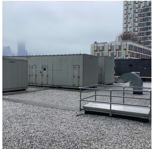
Roof 1 - North view
