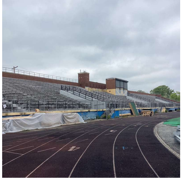
Facade A - Northwest view
