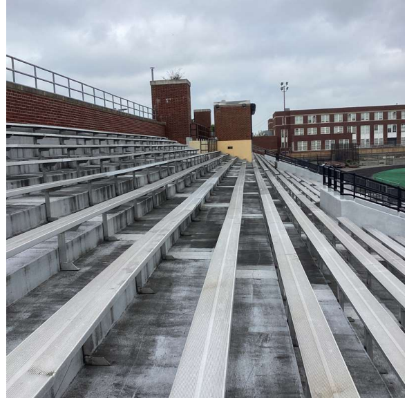
Roof 1 - Northwest view
