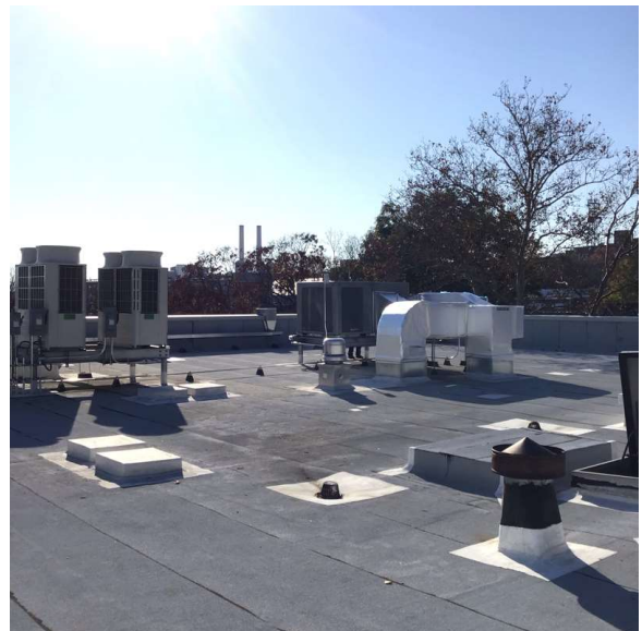
Roof 1 - Northwest View
