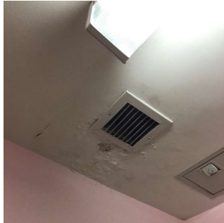
Roof 1 - Room 301C
