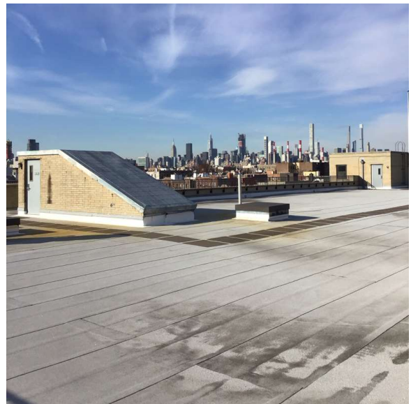
Roof 1 - East View
