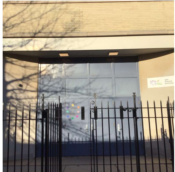
Facade A - 37th Street
