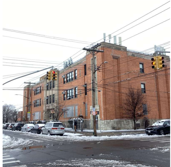
Corner 111th Avenue and 128th Street - North view
