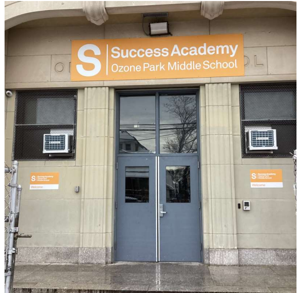
Facade A - 128th Street
