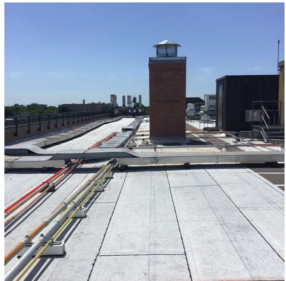
Roof 1 - South view
