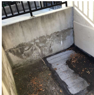
Facade C No violations recorded.
