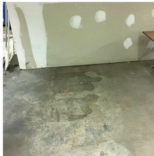
Roof 1 - Basement Elevator Shaft No violations recorded.
