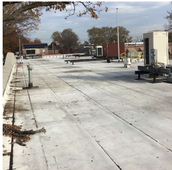
Roof 1 - West View
