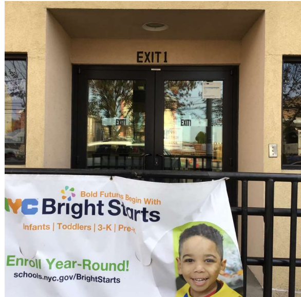
Facade A - 23rd Avenue
