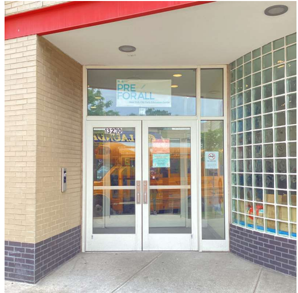
Facade A - Jamaica Avenue
