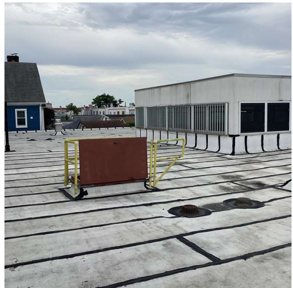
Roof 1 - North View
