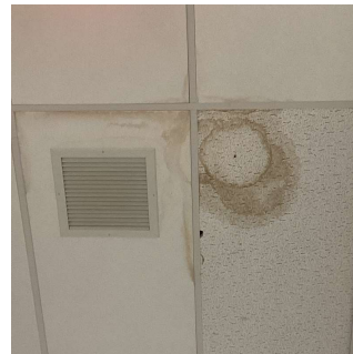
Roof 1 - Corridor near Room 108 No violations recorded.
