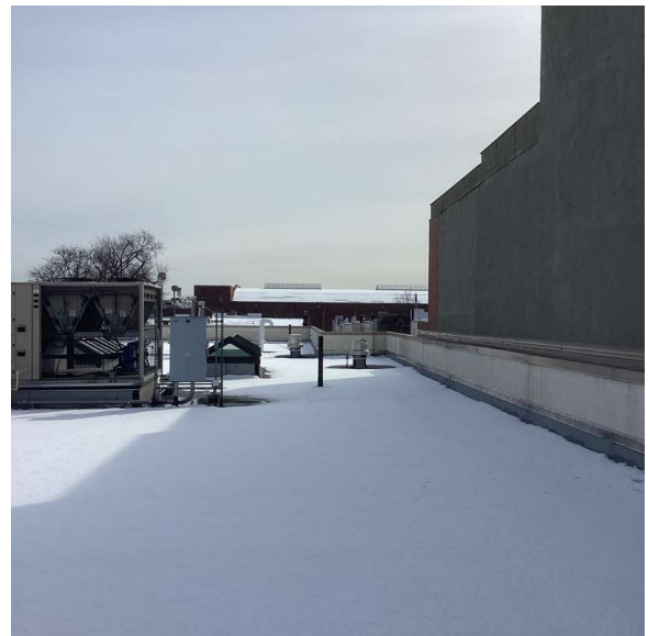
Roof 1 - South view
