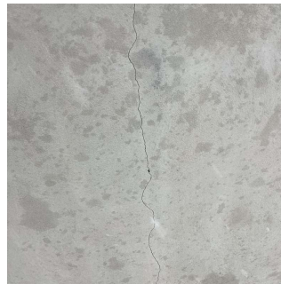
Roof 1 No violations recorded.
