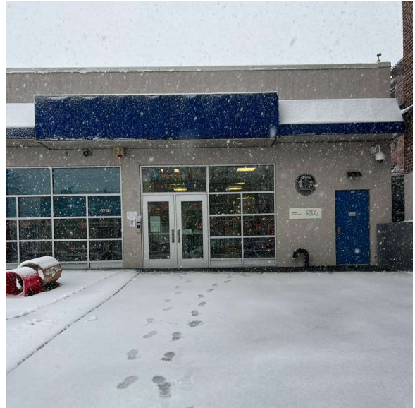
Facade A - 76th Street
