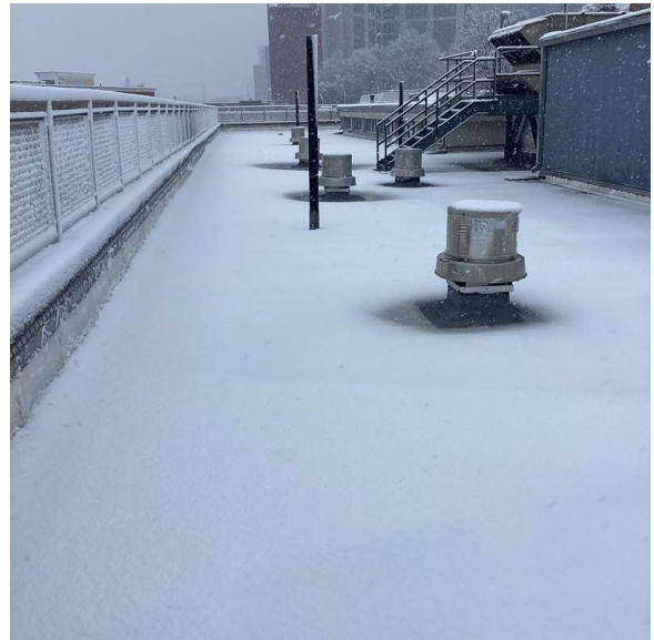
Roof 1 - Southwest View
