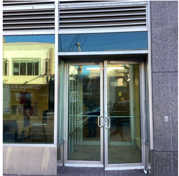
Facade A - Jamaica Avenue
