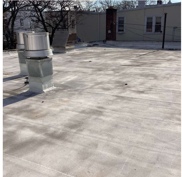
Roof 1 - Southeast View
