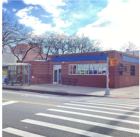
Corner of Corona Avenue and 104th Street - Southwest View
