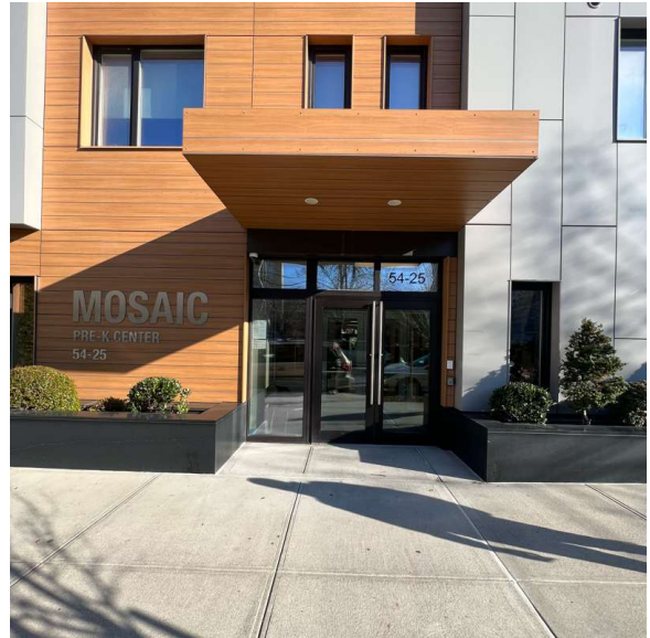
Facade A - 101st Street
