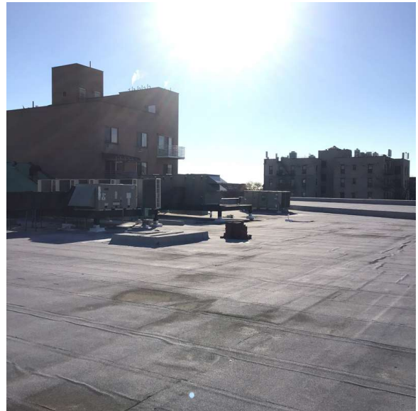
Roof 1 - South view
