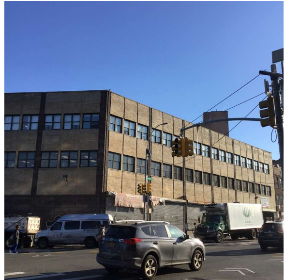
Corner of Broadway and 75th Street- Northeast view
