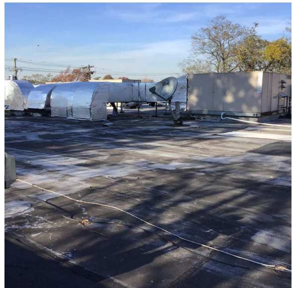
Roof 1 - North view
