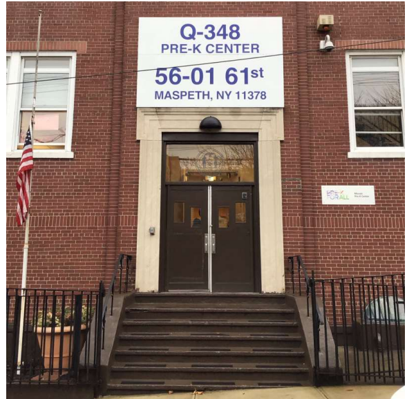
Facade A - 61st Street
