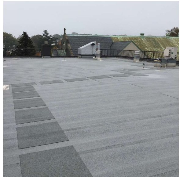
Roof 1 - Southwest View
