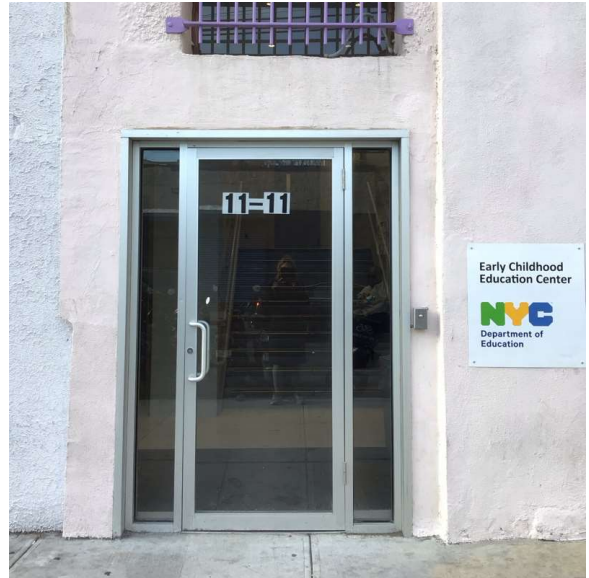
Facade A - 12th Street
