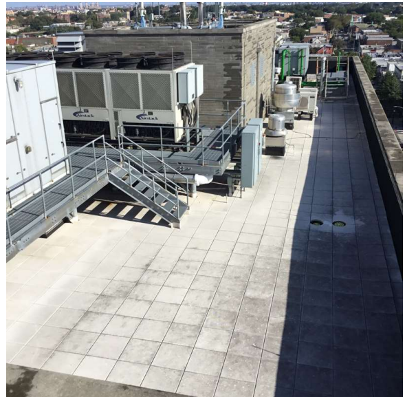
Roof 1 - North View
