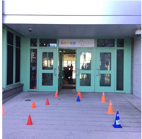
Facade A - 57th Street
