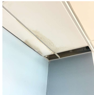
Roof 1 - Room 502 No violations recorded.
