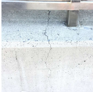
Facade A - HC Ramp No violations recorded.
