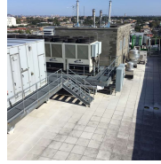
Roof 1 - North View
