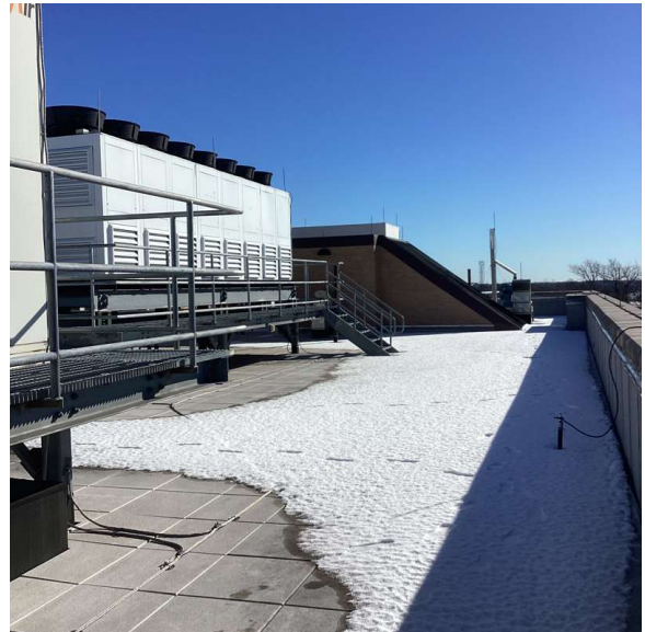
Roof 1 - Northeast view
