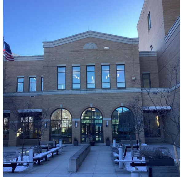
Facade A - Raleigh Street
