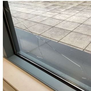
Facade A - 4th floor corridor near Rooms 401A, 401, 403
