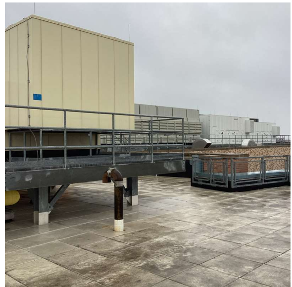
Roof 1 - Northeast View
