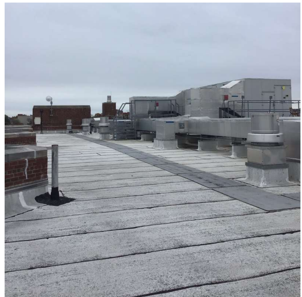
Roof 1 - Southwest View
