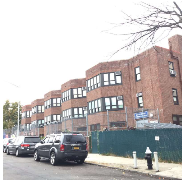
97th Street - Southwest View
