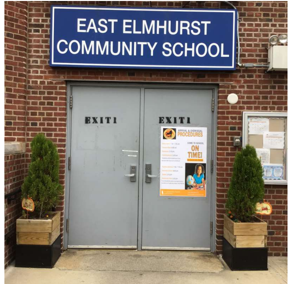
Facade A - 97th Street
