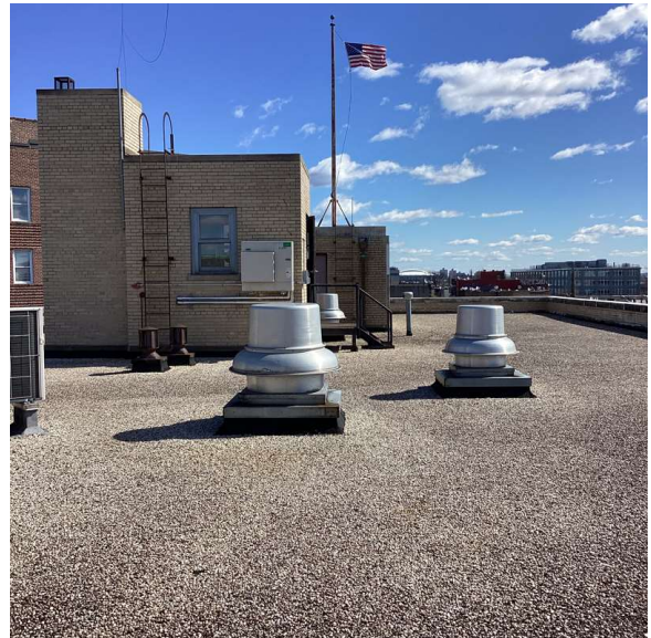
Roof 1 - Northeast View
