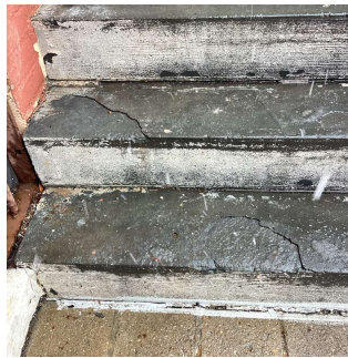
Facade C No violations recorded.
