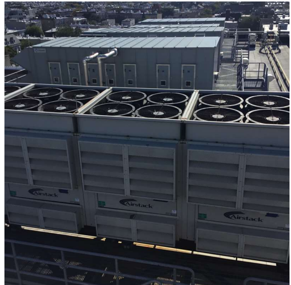
Roof 1 - Southeast View
