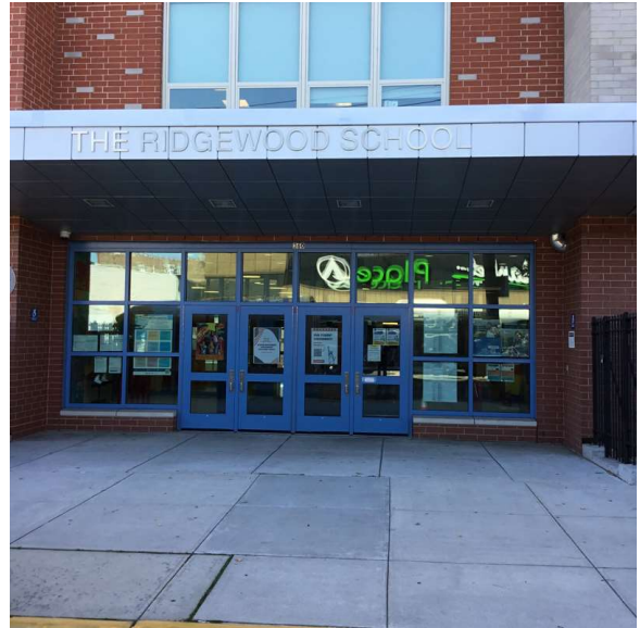
Facade A - Seneca Avenue
