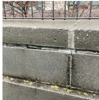
Roof 6 - Facade L
