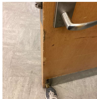
Entrance From Cafeteria near Exit 7
