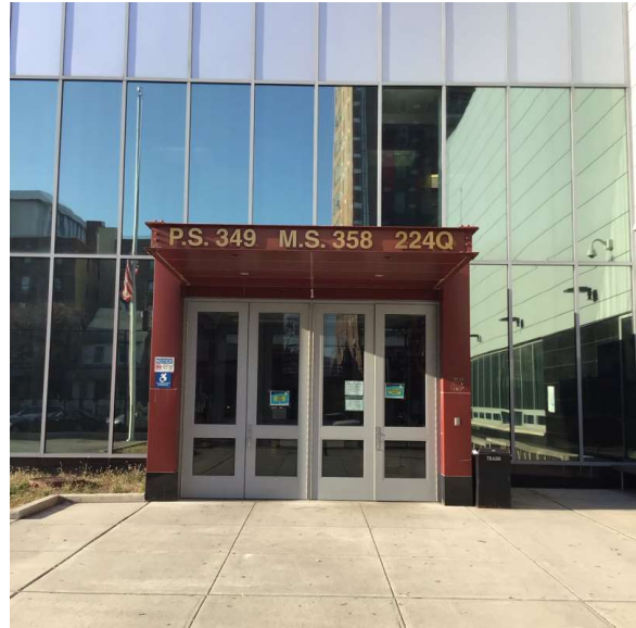
Facade A - 164th Street
