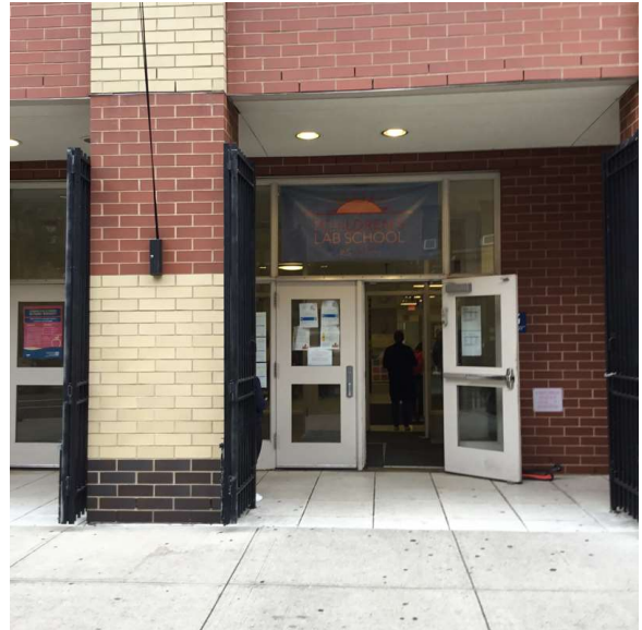
Facade A - 42nd Street
