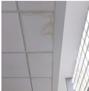
Facade G - 5th Floor Corridor near Elevator (Facade G - 4th, 3rd, and 2nd Floor Corridors near Elevator
